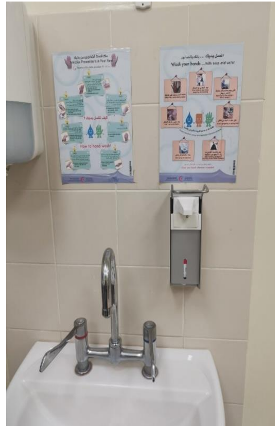
Figure 20: A handwashing basin with instruction posters at a healthcare facility in Oman
