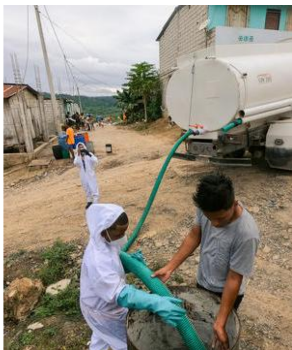
Pit emptying Ecuador (UNICEF 2021)
