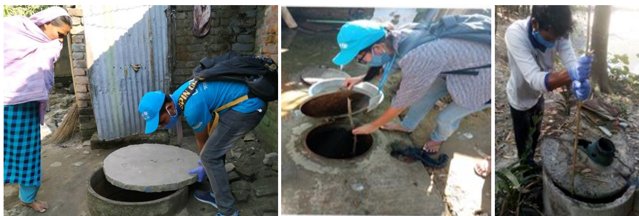
Box 6. Sanitary inspection – opening the containment
