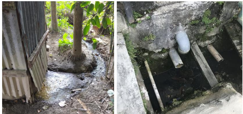
Figure 6. Overflowing pit in Bangladesh and pit discharging to drain in Indonesia viii
