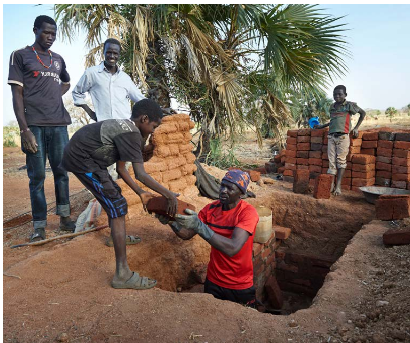
With help from his son, a man digs a pit for sanitary latrine near his house in Tellou Aljouba village, 6 km East of the town of Kadugli, in South Kordofan province. Sudan.
